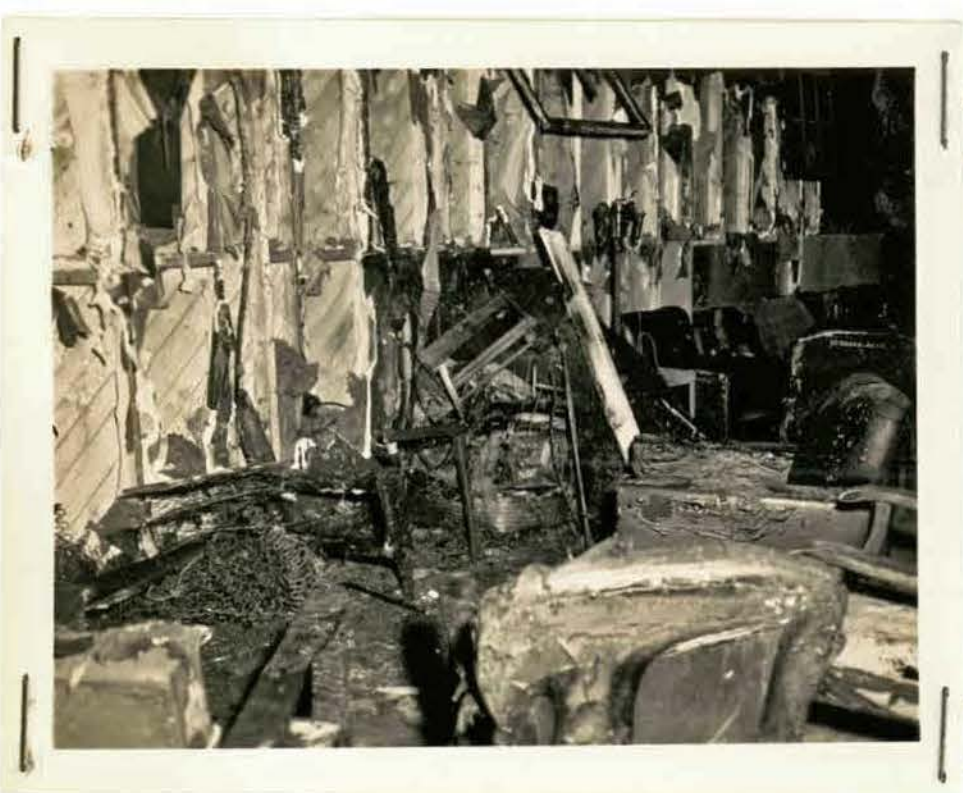
Neg. No DB 7745 Dispo: L HQ Dest Photo'g Manuel Dept FIRE HALL Caption SHIPS COMPANY MESS FIRE View of damage to the interior of the lounge
