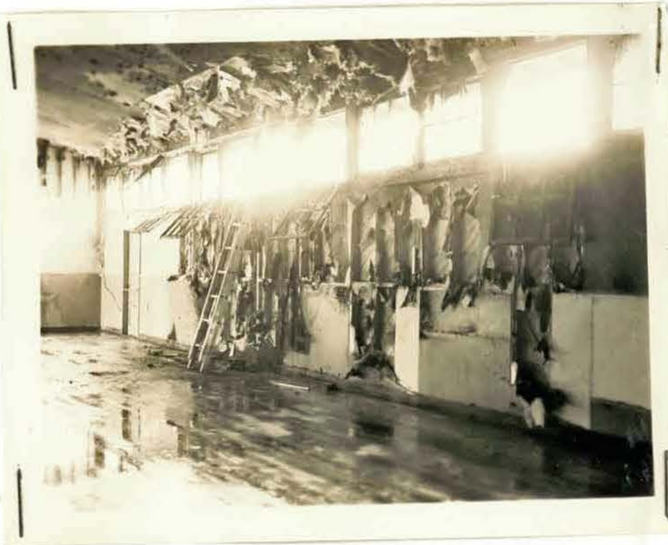
Neg. No DB 7747 Dispo: L HQ Dest Photo'g Manuel Dept FIRE HALL Caption SHIPS COMPANY MESS FIRE View of damage to the interior of the lounge.
