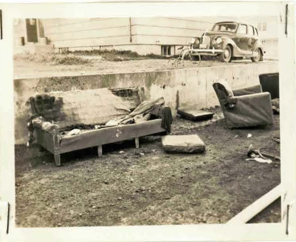
Neg. No DB 7748 Dispo: L HQ Dest Photo'g Manuel Dept FIRE HALL Caption SHIPS COMPANY MESS FIRE View of damaged furniture placed on driveway beside the Mess.
