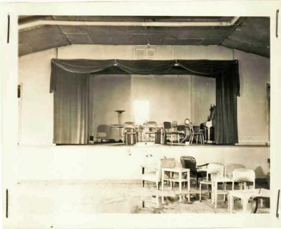
Neg. No DB7746 Dispo: L HQ Dest Photo'g Manuel Dept FIRE HALL Caption SHIPS COMPANY MESS FIRE View showing damage to the interior of the lounge.
