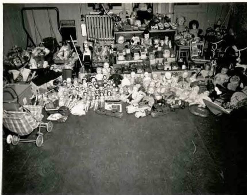
Neg. No. DB 8222 Dispo: L HQ Dest Photo's Arndt Dept Fire Dept. Caption Xmas Parade View of toys which were collected by the Fire Dept., repaired to be given to the needy children
