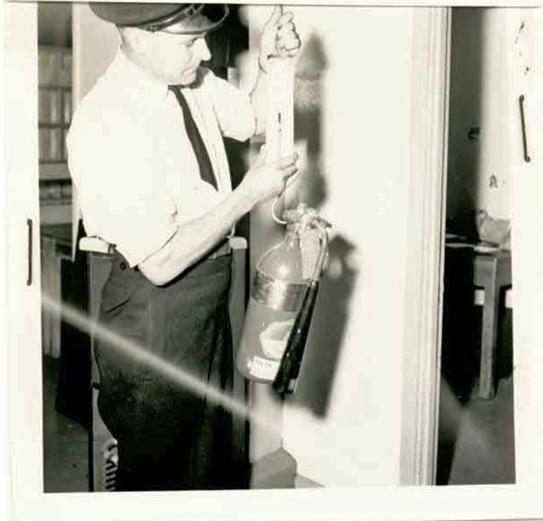
DB: 9137 ✓ Dispos: 1 HQ Dest. Photog: ELLIS Dept. Fireman O. Belliveau checking fire extinguisher for correct weight.
