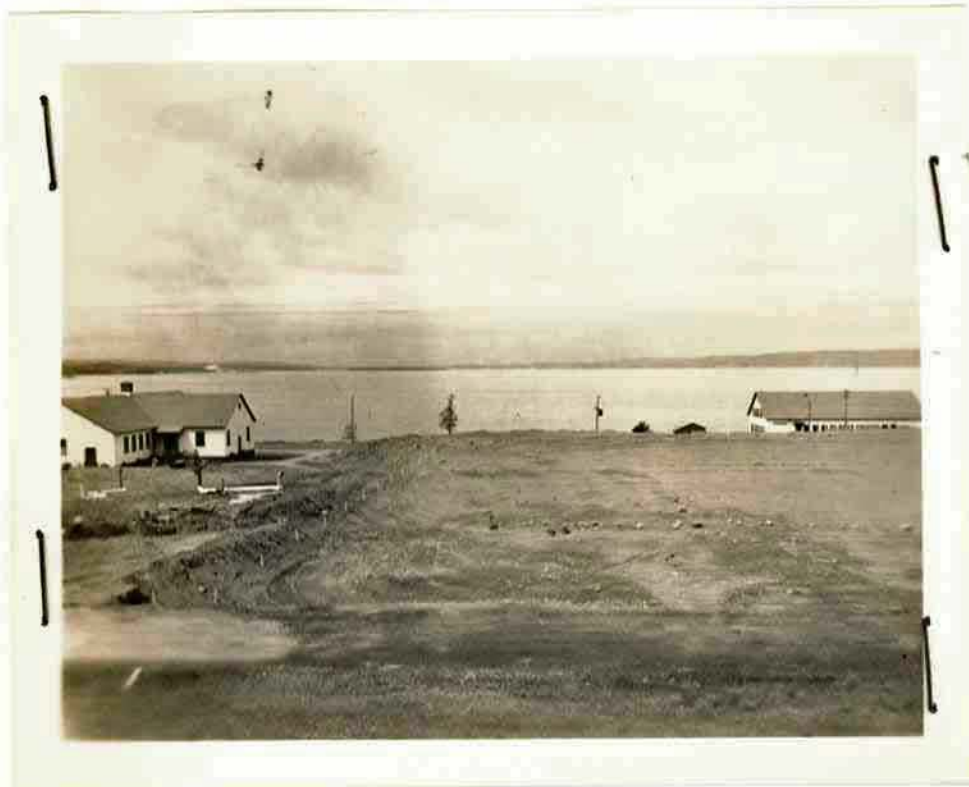
DB: 9231 DISP: W HQ Dest. Photog: MANUEL Dept: Maintenance Progress photo of new Sports Field, looking west from Wardroom
