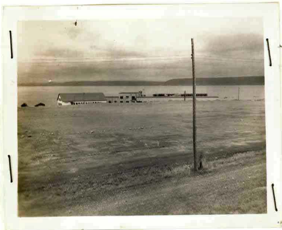
DB: 9232 Disp: W HQ Dest. Photog: MANUEL Dept: PA&T Progress photo of new Sports Field looking west from Wardroom
