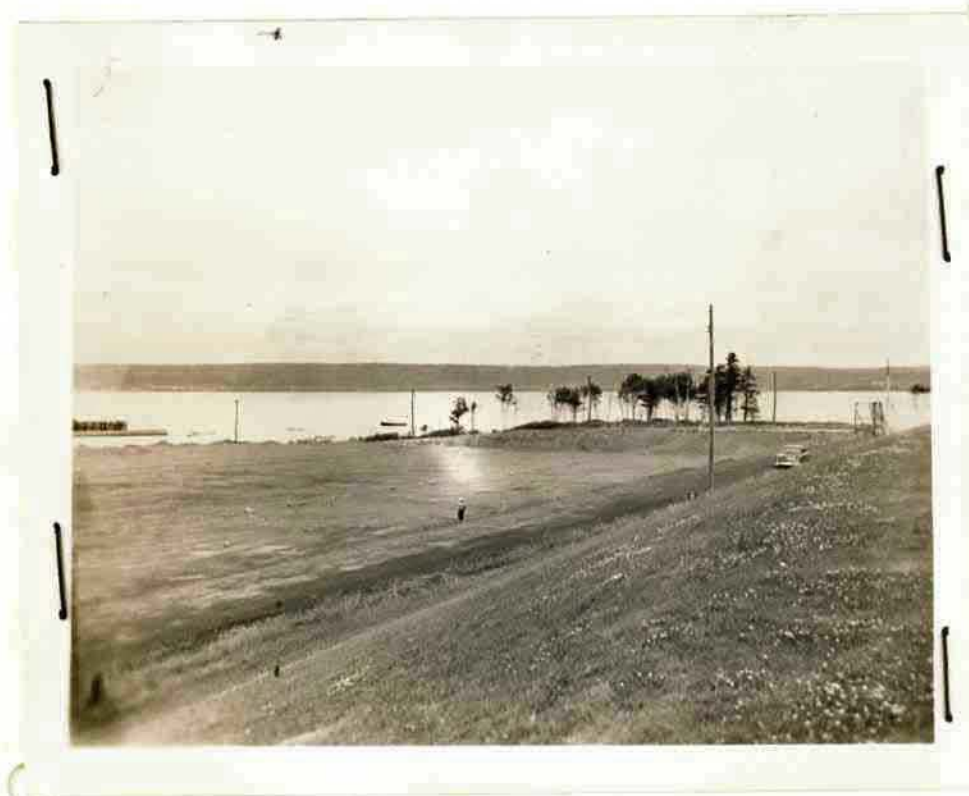
DB: 9233 Disp: W HQ Dest. Photog: MANUEL Dept. Maintenance Progress photo of new sports field loking west from Wardroom.
