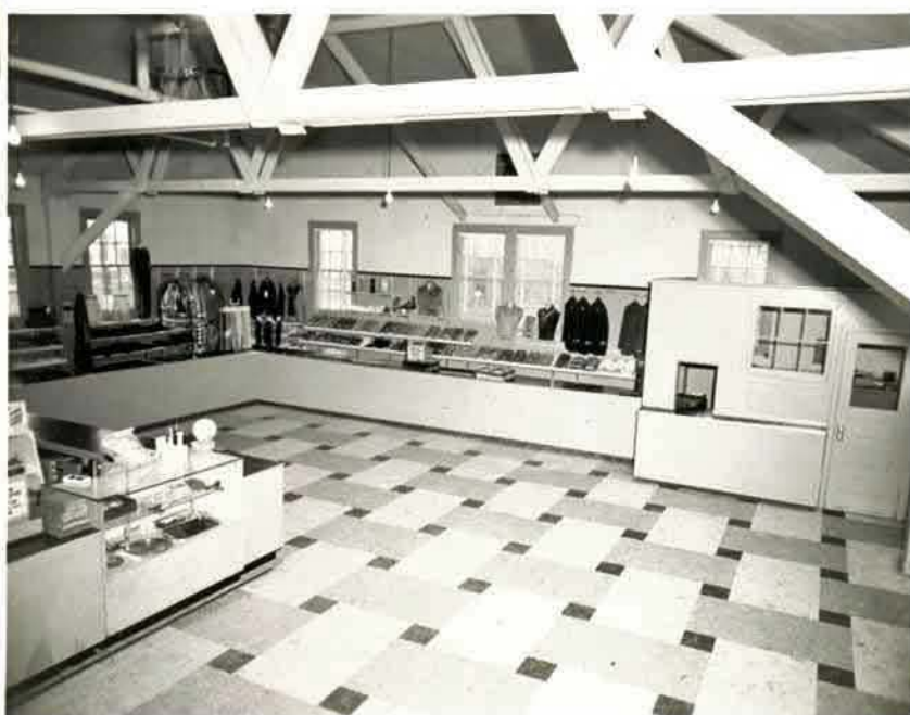
Interior of Central Canteen
