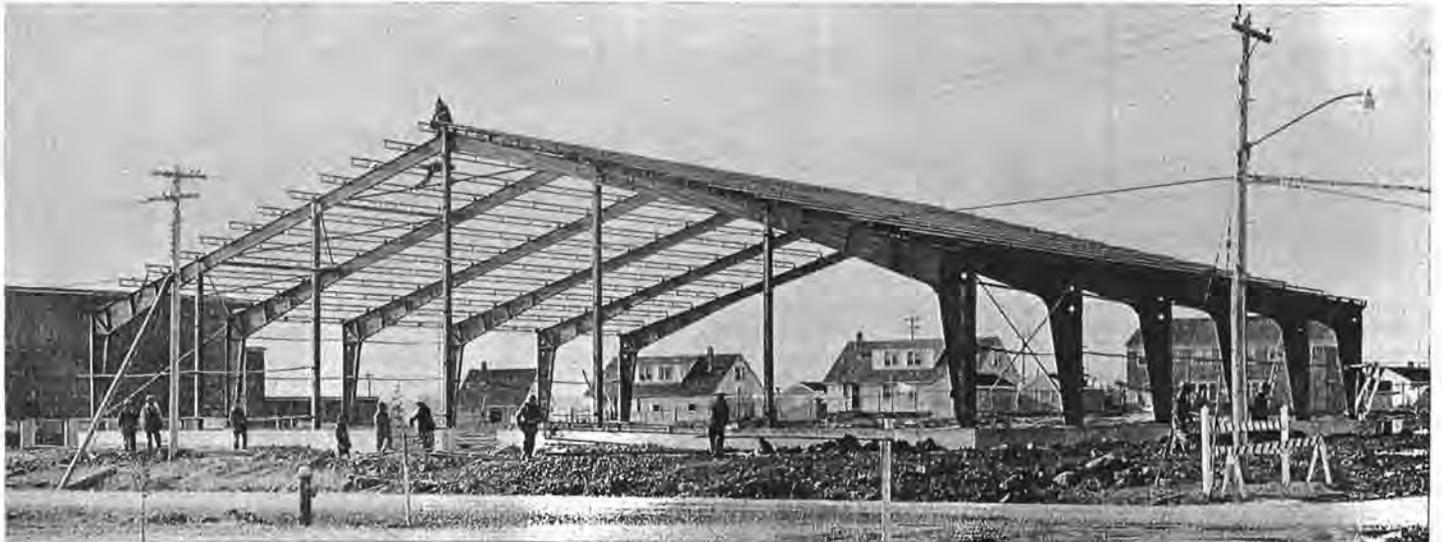
Half of the main beams were already in place when this picture of the ice rink being built at HMCS *Shearwater* was taken on January 23. A non-public fund venture, the rink is adjacent to the gymnasium, part of which is shown on the left. (DNS-30238)
