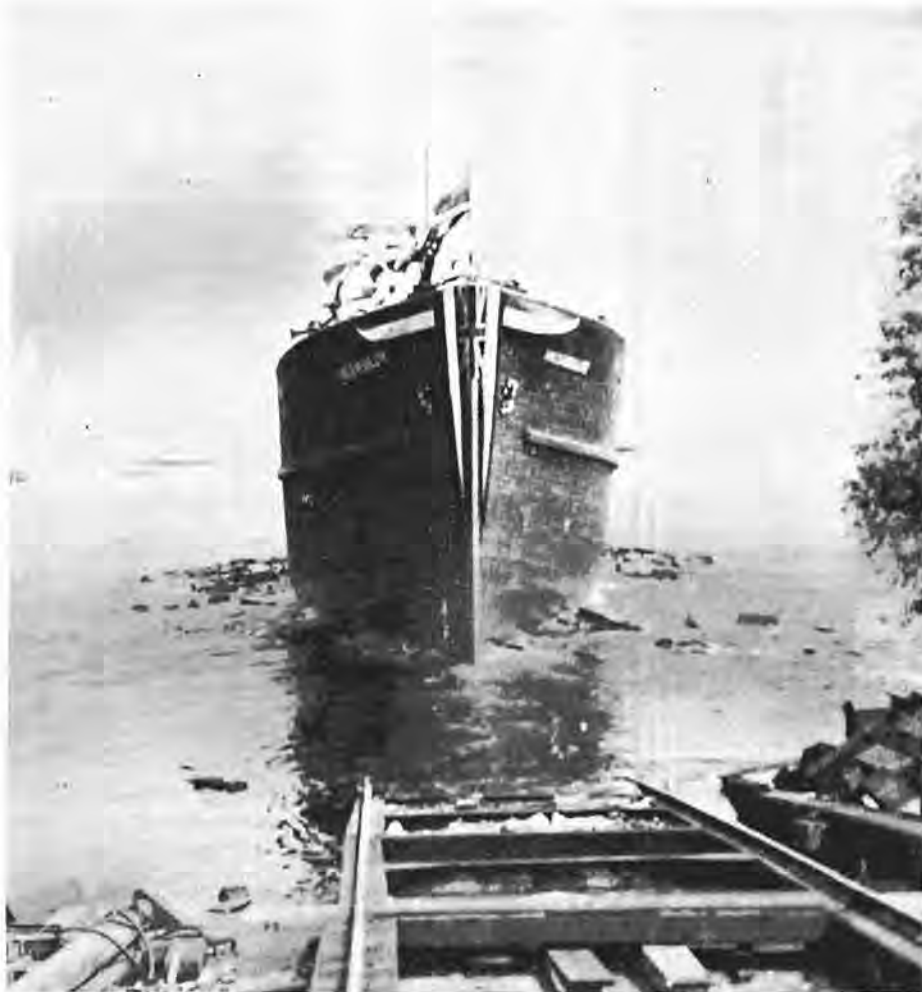
HMCS "Resolute", tenth ship of her class to be launched, slid down the ways in a marine-railway launch at the Canadian Shipbuilding and Engineering Company yard in Kingston, Ont., Saturday, June 20. Mrs. T. R. McLagan, wife of the president and general manager of Canada Steamship lines, pronounced the traditional words. (O-1588)
