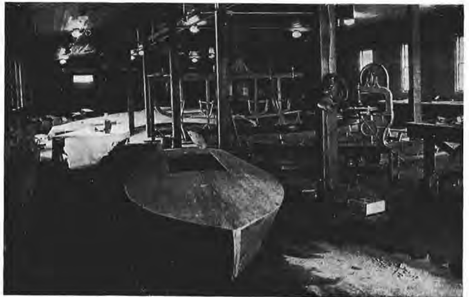
Snipe class boats in various stages of construction in the RCN Yacht Club's new shop on the jetty at "Naden". When the boats are near completion, lots are drawn to determine ownership and the owners finish off their boats before putting them in the water. (E-11088.)
