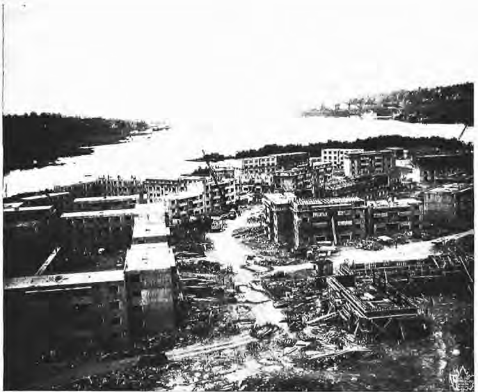
A new community is springing up on the shores of Tufts Cove, across the harbour from the North End of Halifax. It is the new naval married quarters project, one of the largest of its kind in Canada. When completed, the Tufts Cove quarters will contain about 1,200 apartment units and will house an estimated 4,000 persons — naval personnel and their families. (DNS-5505).
