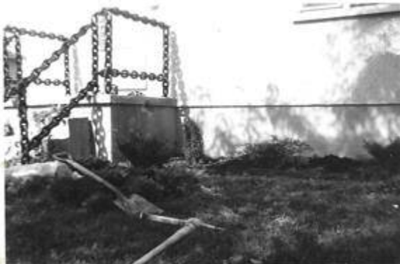
Some chain attached to the anchor was used to create stair railing at front of home.
