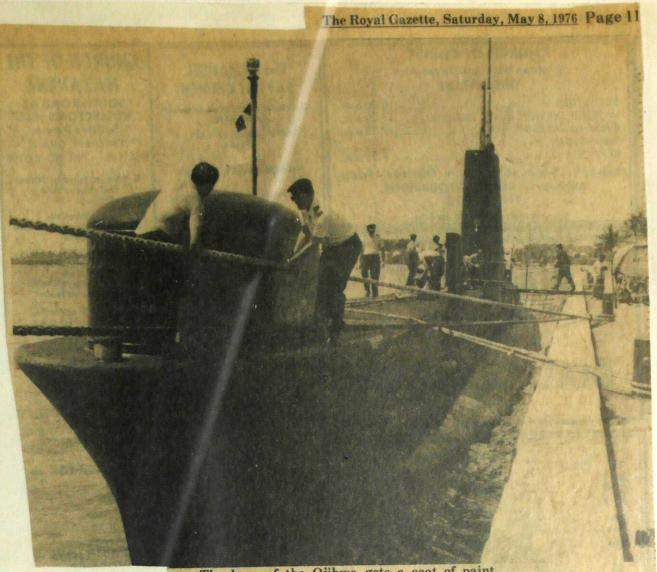
The bow of the Ojibwa gets a coat of paint. Much of the 'sub's' outer surfaces are fibreglass to reduce maintenance work.
