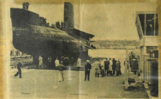
HMCS OJIBWA, weighing a mere 1,600 tons, became the first vessel yesterday to be lifted ashore by Halifax Dockyard's new \$5,000,000 syncrolift. The lift has a capacity of 4,000 tons — 6,200 tons including the platform apparatus — and took two years to install. The Ojibwa, Canada's first submarine, is in for a reflic which is expected to take about a year to complete.
