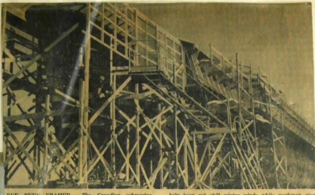
I'VE BEEN FRAMED — The Canadian submarine Ojibwa has almost disappeared behind a network of wooden cribwork erected along the sub's bulky hull to
