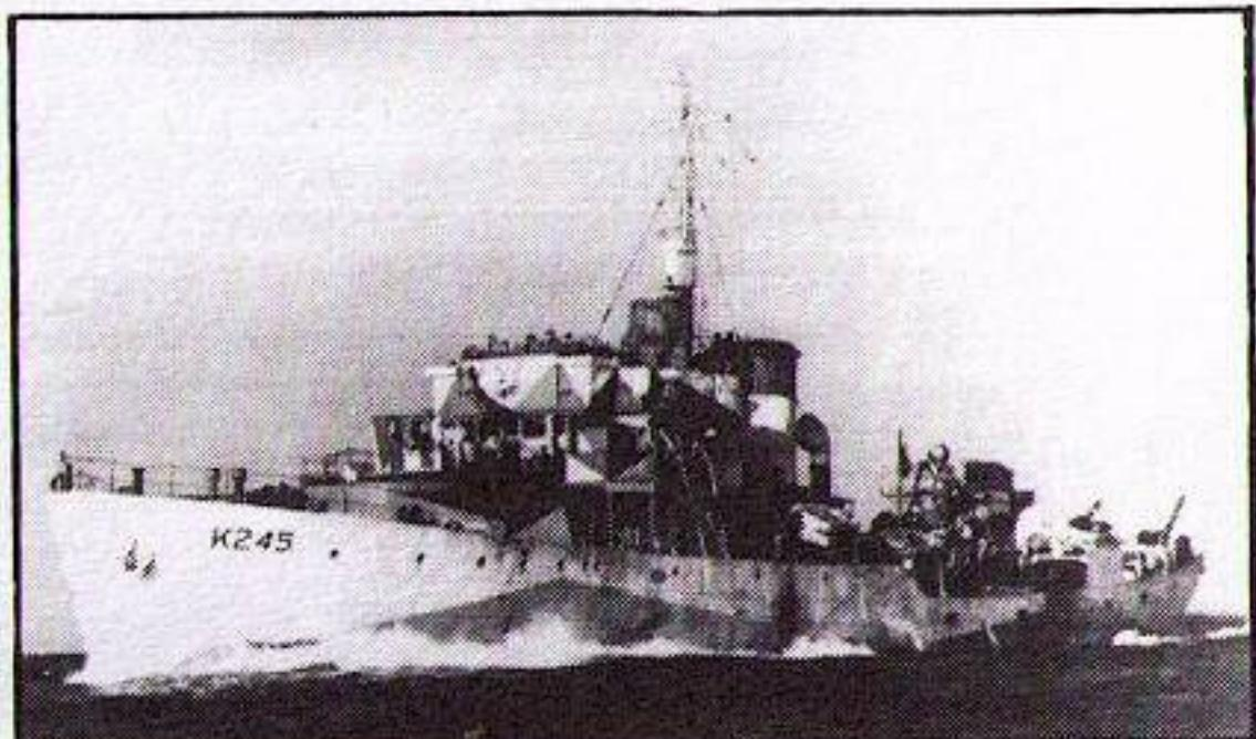
With a length overall of 208 feet, a beam of 33 feet and drawing 13 feet of water, FREDERICTON was originally designed as a costal vessel and not a 'blue water ship'. Driven by the increased successes of the German U-boat campaign however, FREDERICTON and other corvettes like her were forced into the ocean escort role and served in this capacity throughout the Second World War.
